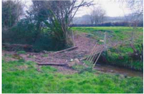
Stream crossing before .....
